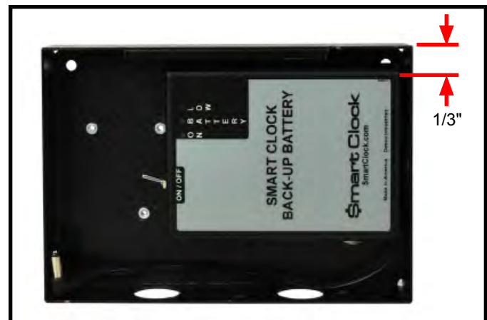
Figure 121. Installing the Smart Clock Back-up Battery into the steel backplate
